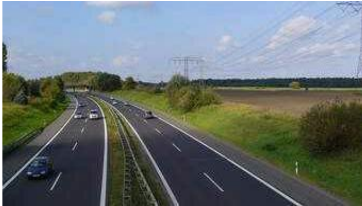
Fig. 1. The asphaltic roads being built by Ikpeazu in Aba (4:42pm on 9 th October, 2015)
