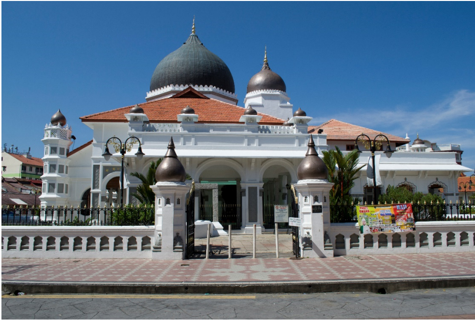
Figure 3. (a) Kapitan Keling Mosque and brick fence (frontal view).
