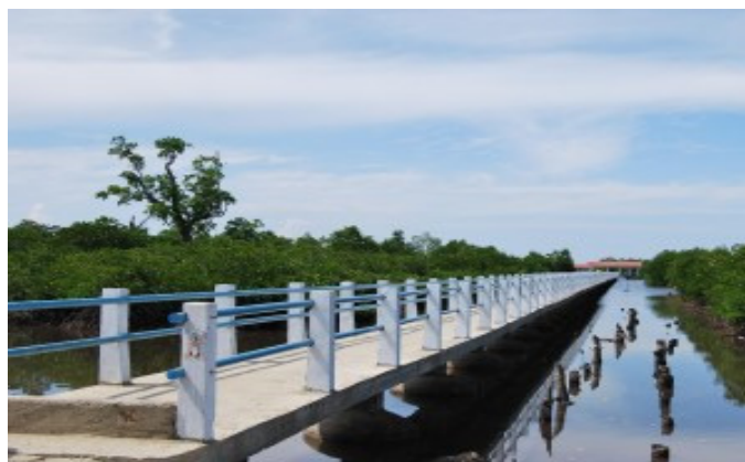
Figure 2. Pedestrian bridge of Torosiaje village
